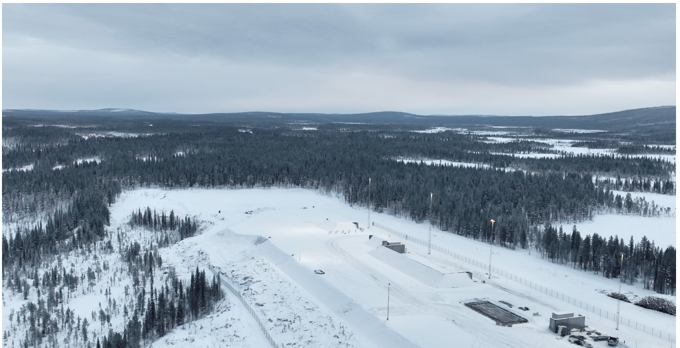
Construction of Spaceport Esrange 2022.
